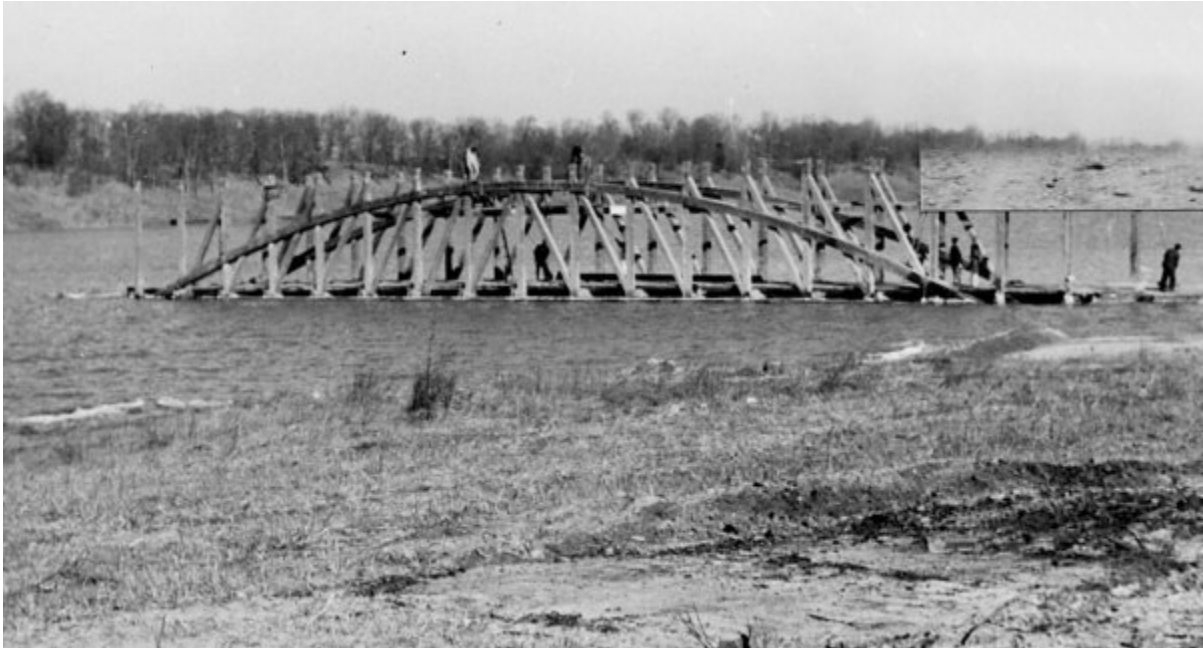
The covered bridge is dismantled
