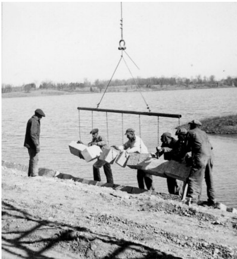
Rip-rap blocks for dam and approaches to bridges
